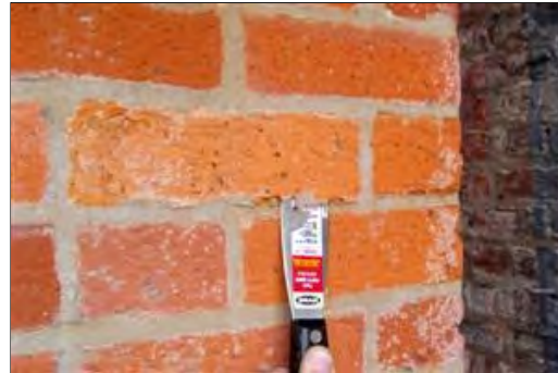
A. Picture 21 Flaking Brick Face
