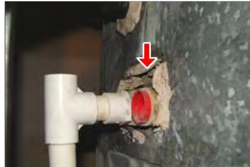
G. Picture 4 Air Gap at Plenum
