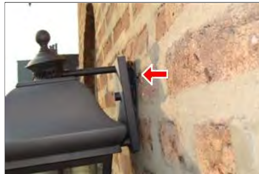
A. Picture 3 South Elevation Light Fixture
