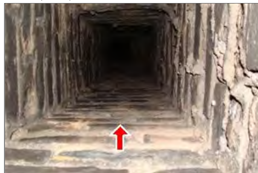
H. Picture 2 South Flue
