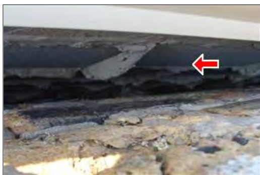
A. Picture 9 Concrete Block Wall at East Elevation
