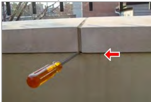
A. Picture 14 Gap at Top of Stucco Finish
