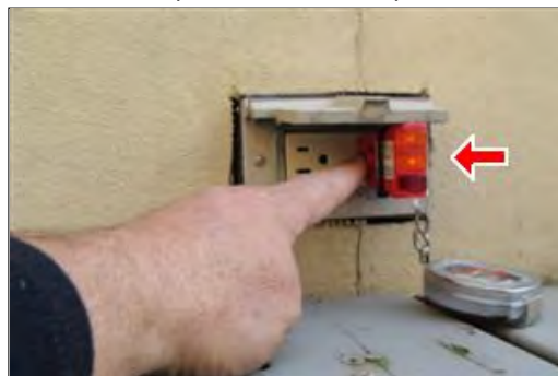
E. Picture 3 Non-GFCI Receptacle at Balcony
